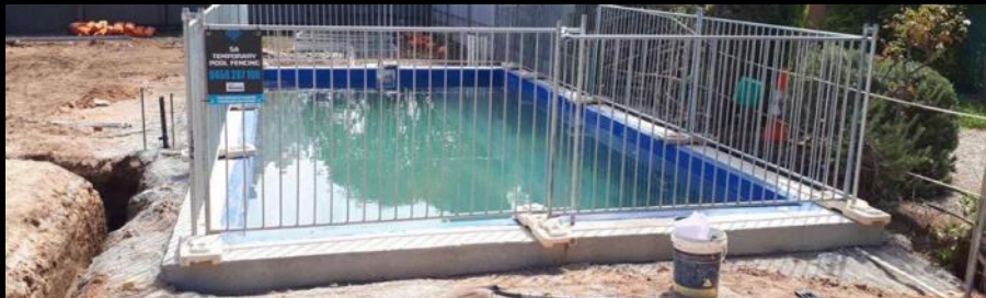
POOL AND CONCRETE BEAM
