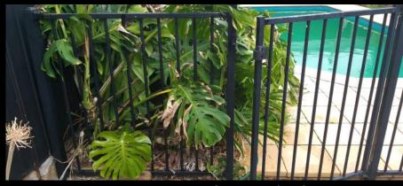
Issues such as gates not self-closing/self-latching can be caused by deteriorated hinges and latches; or by obstructions such as over grown shrubs. These areas are quickly identified and solutions provided.
